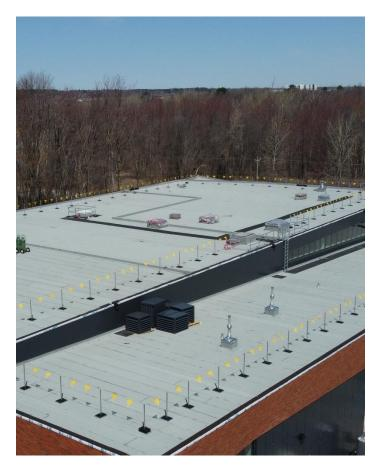
The Millenium freestanding warning line is used to delimit areas on roofs to allow work and traffic in full compliance with provincial regulations\* regarding the prevention of falls from heights.
